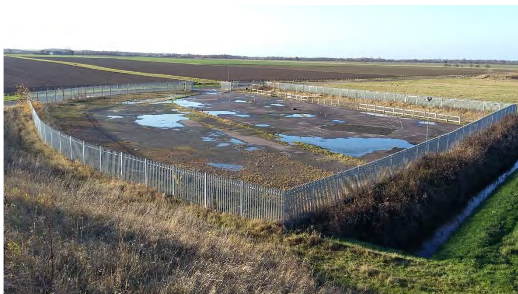
Figure 1: The Site at present
